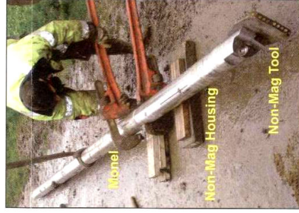
Installing non-mag housing, containing SST® transmitter, and monel on tool
